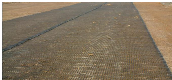
Fig.4. Laying Scene Diagram of Geotechnical Grille
