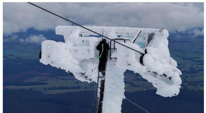
Figure 2. Ice on Gondola support tower, Mt Ruapehu [14]
