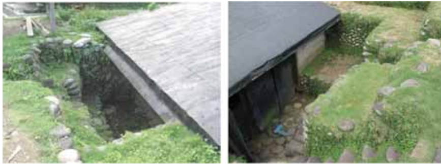
Figure 17: The different pit depths of a main house in Yehyin (left-hand side) and Langdau (right-hand side).
