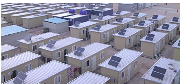
Figure 3. Containers used as temporary houses [11]
