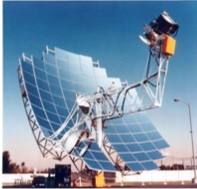
Fig. 1 – Example of Dish-Stirling solar concentration system.
